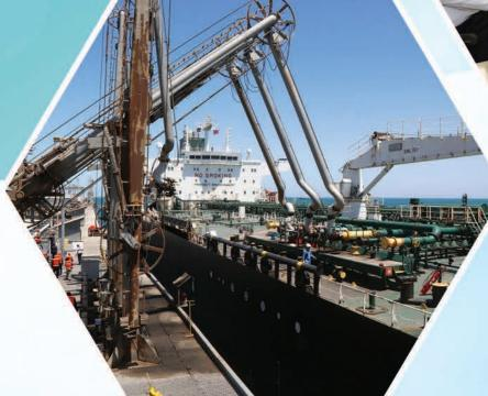
At the last stage, crude oil enters the tanker through the loading arms mounted on export quays.
